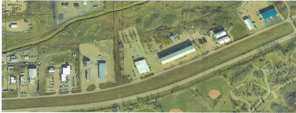
North Signage Corridor
